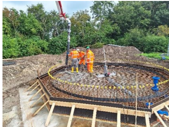
Fundering slibbuffertank te Olst
